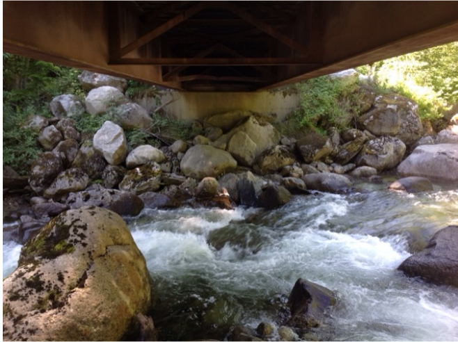
Right Bank Abutment when facing downstream
