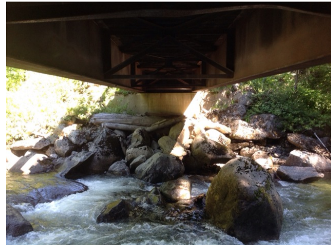
Left Bank Abutment when facing downstream
