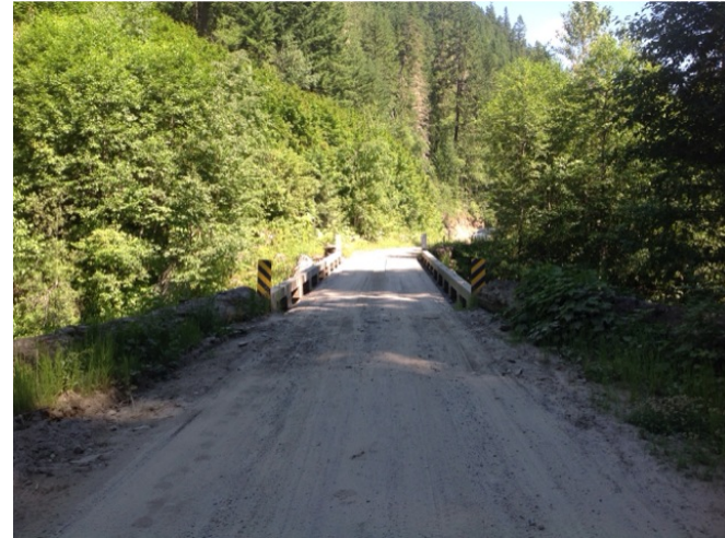
Approach from Right Bank when facing downstream
